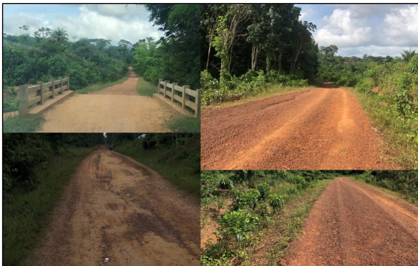
Figure 7: Road sections of feeder roads in Bong county, Liberia
